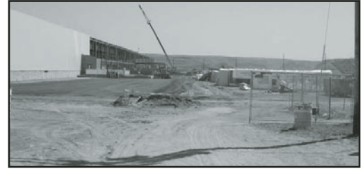
Early construction of the Railex facility in Wallula.
