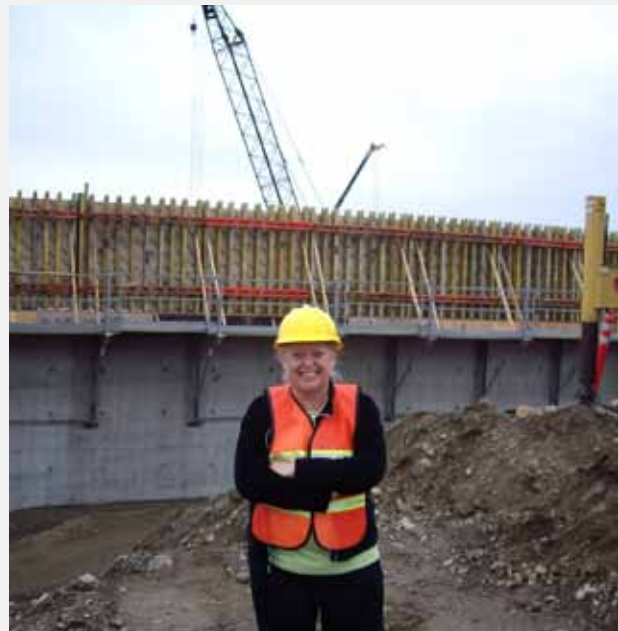
FMSIB Executive Director, Karen Schmidt, tracking progress on a FMSIB construction project
