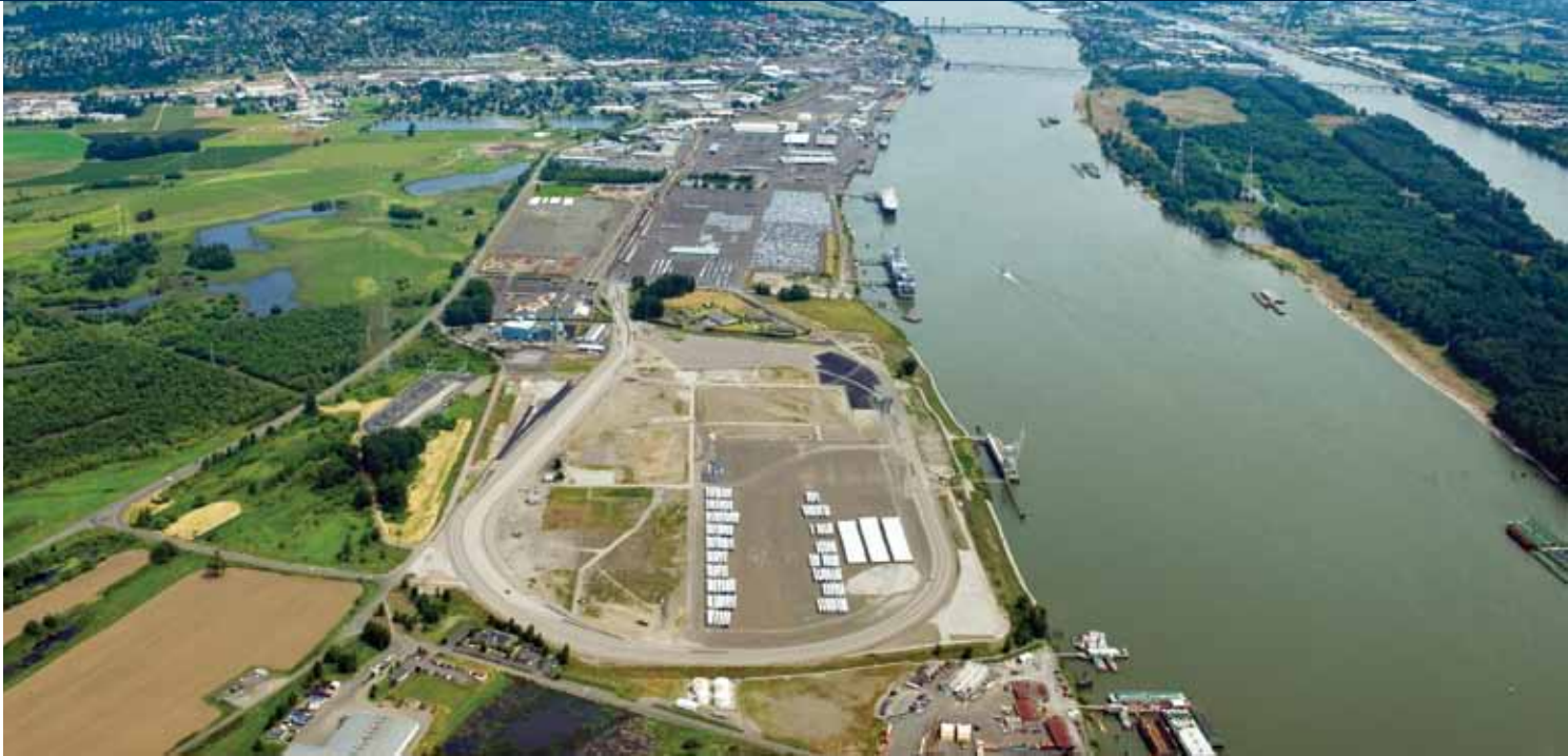
Port of Vancouver, West Vancouver Freight Access Project, Phase 2, loop track, completed in 2010
