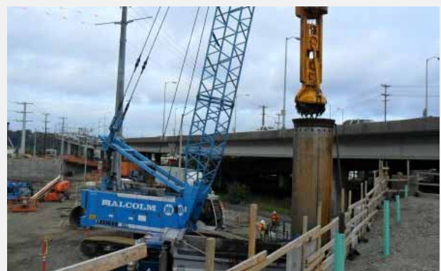
Construction activity on East Marginal Way, photo courtesy of Port of Seattle
