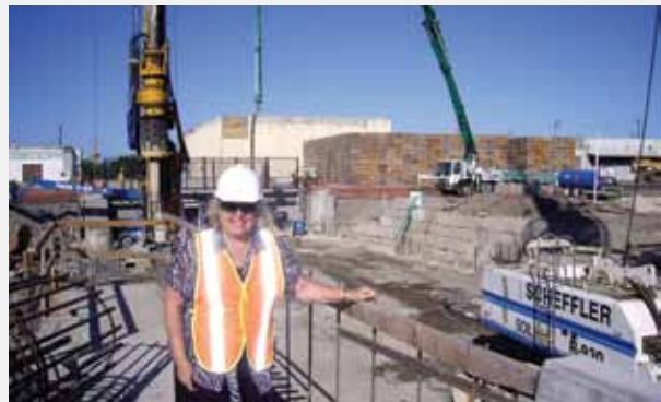
Bob Desgrosellier, City of Yakima, Senior Engineer and Karen Schmidt, FMSIB Executive Director, observing construction of the Lincoln Avenue/BNSF undercrossing in downtown Yakima
