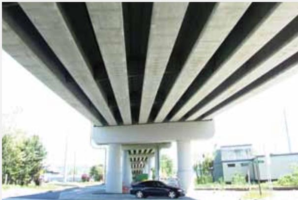
Lincoln Avenue Grade Separation, Port of Tacoma
