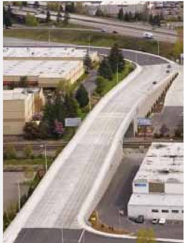
City of Kent, 228th Street and BNSF Rail Grade Separation
