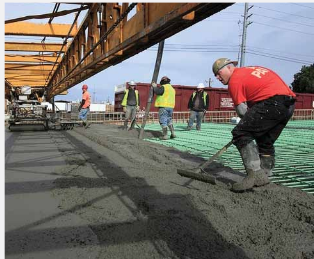
Lincoln Avenue Construction, Port of Tacoma
