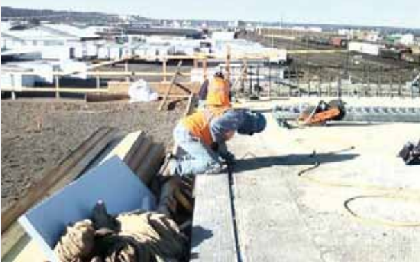
City of Spokane, Havana Street Construction
