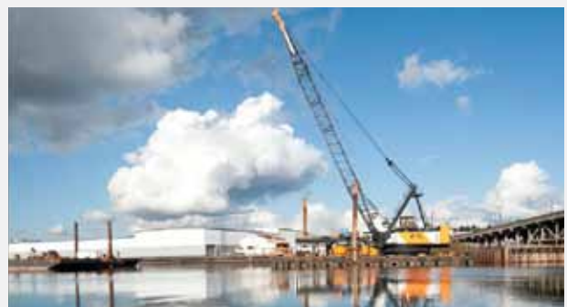
Construction photos of South Park Bridge, fall 2011 Photo credit: John Stamets
