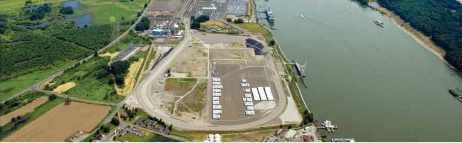
Port of Vancouver USA, West Vancouver Freight Access Rail Project, Loop Track
