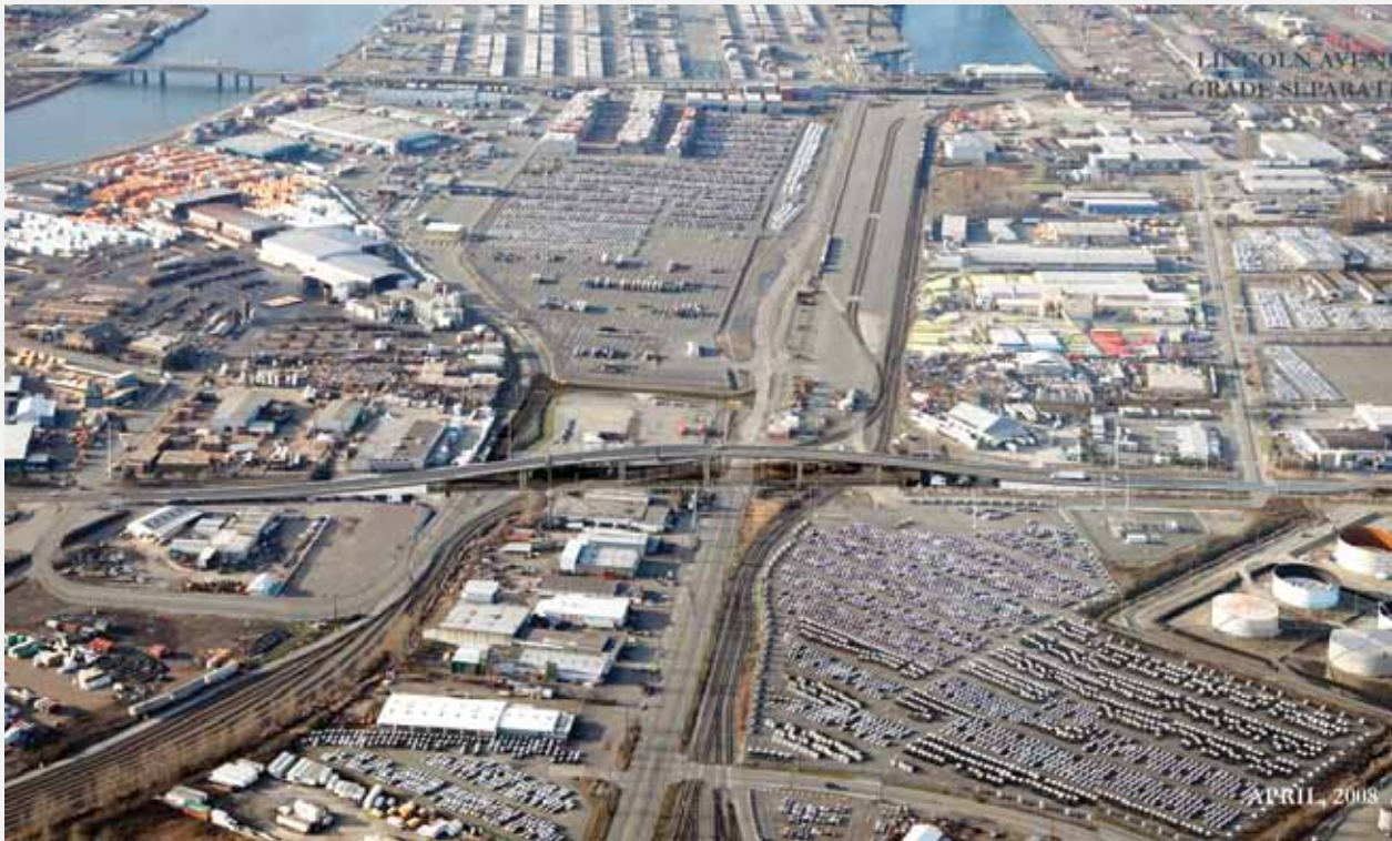
Lincoln Avenue Grade Separation, Port of Tacoma
