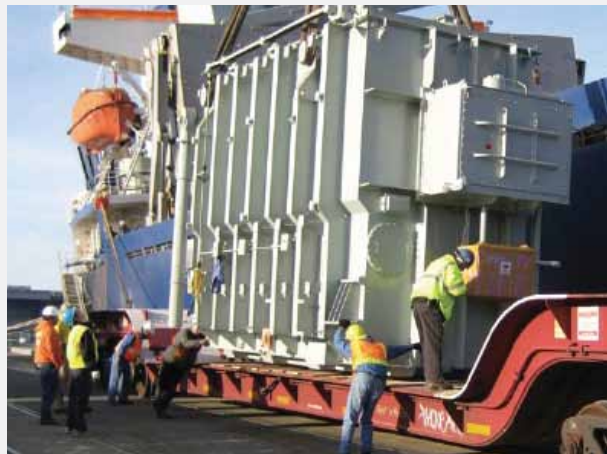
Port of Everett, Loading Generator Parts
