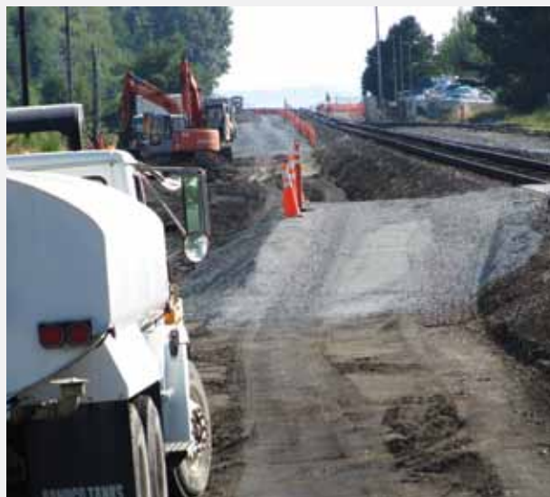
BNSF Track Construction, Summer 2011
