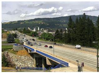
This project was completed in September of 2017. Built in 1951, the Sullivan Road Bridge was rated as structurally deficient in 2009. It is a critical transportation link that connects industrial areas north of Spokane and in Spokane Valley with I-90. The project replaces the existing 2-lane bridge with a new 4-lane bridge. The structure carries about 26,000 vehicles per day and has a truck volume of about 24 percent. The new bridge allows weight restrictions on the route to be lifted.
