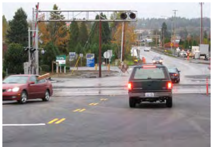
Phase I of the SR 202 improvement was completed in October, 2007.
