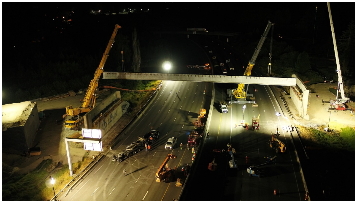
Figure 1 - Nighttime placement of bridge girders spanning I-5, 70th Ave. E. Undercrossing (August 2020)
