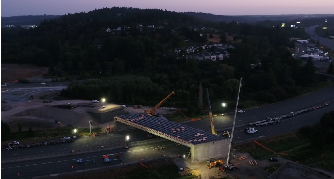
Figure 2 - Completed placement of bridge girders, 70th Ave E. undercrossing (August 2020)
