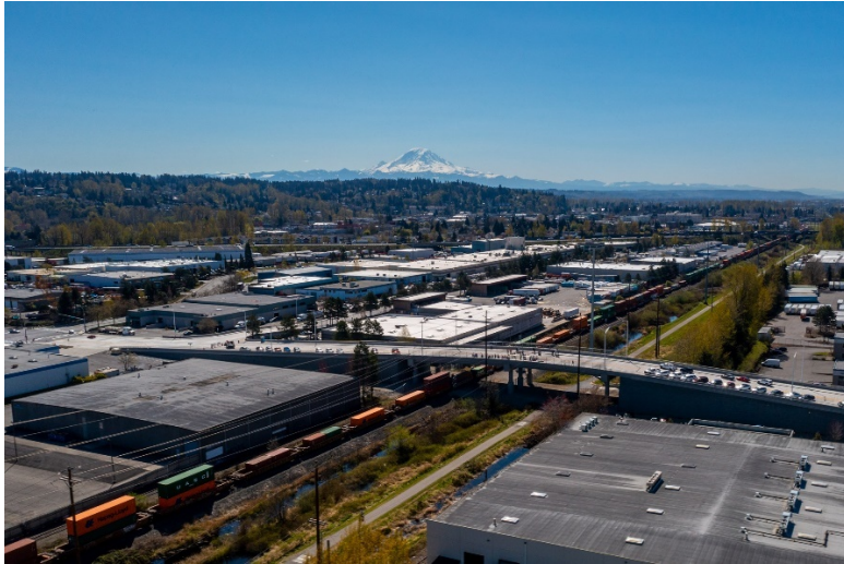
Figure 2 - City of Kent, South 228th Grade Separation (UPRR), looking southeast
