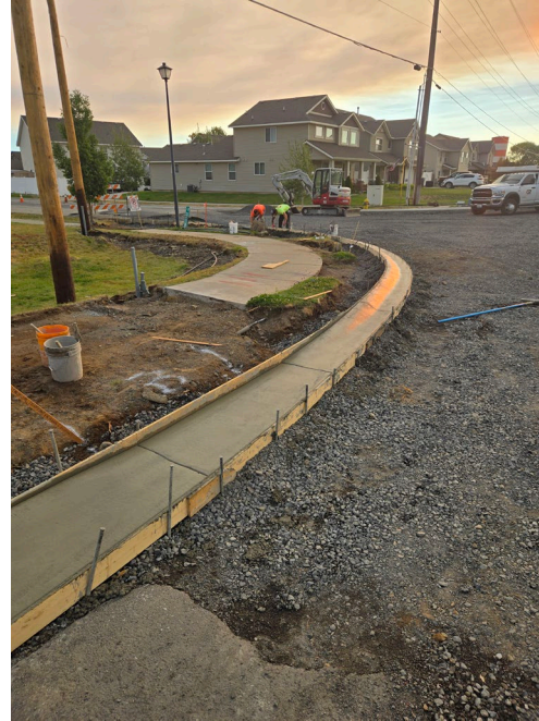
Grade prep work for paving
