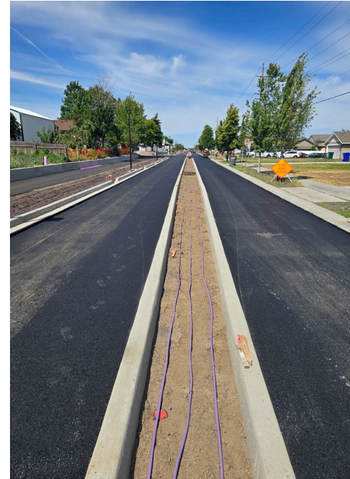
Grade prep work for paving
